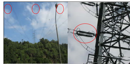
Fig. 1. Three OHGW and 22 pieces porcelain insulator
